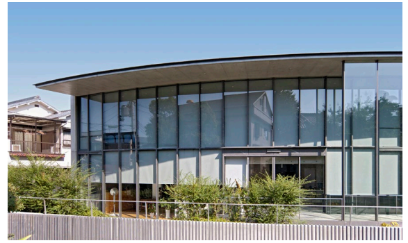
Although interior blinds and light-coloured curtains behind the windows can reduce reflections, they often still occur. Such measures cannot be expected to provide effective protection against collisions, especially as blinds are not permanently closed.
