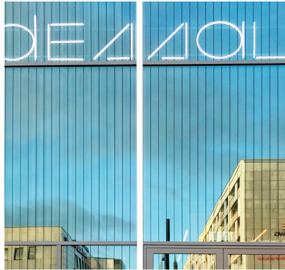
To prevent bird collisions at the new Bauhaus Museum in Dessau, Germany, more than 2700m 2 of glass façade were retrofitted with a plotted line pattern.
