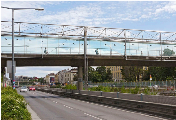
Glass windbreaks on bridges and connecting walkways are among the most conspicuous traps for birds. In many places, silhouettes of birds of prey have been stuck onto the glass. While these are ineffective, they confirm that collisions occur on these areas.
