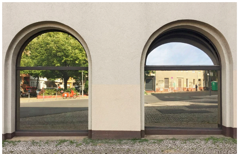
Reflective sun protection films create realistic mirror images. To birds, these windows look like arches they can fly through.
