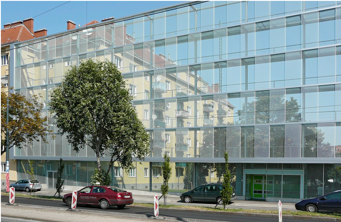
The bird protection pattern used in this noise barrier by Treusch architecture in Theodor-Körner-Hof in Vienna deliberately emphasises its three-dimensional structure.
