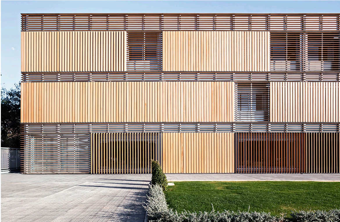
In the west block of the Centre d'Idiomes de la Universitat de València, Spain, by Arkitera SLP, the combination of fixed and movable sunshade slats defines the structure of the façade.
