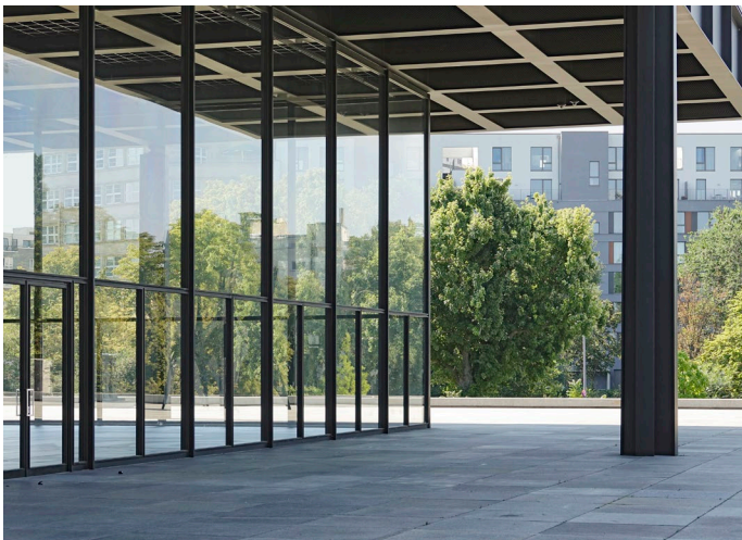
Transparency and openness as the epitome of modernity characterise the architecture of this art gallery, the Neue Nationalgalerie, in Berlin. For birds, the unobstructed view through the glass building becomes a deadly trap.
