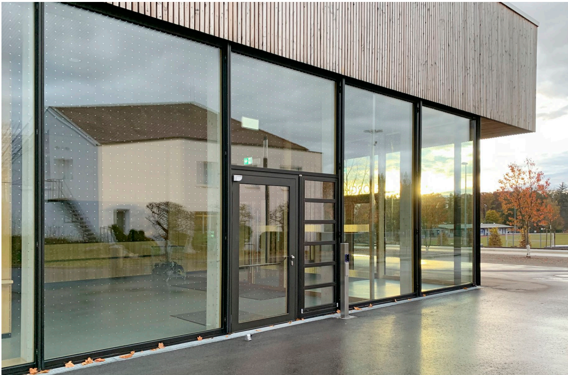
This grid of 9 mm metallic dots at 90 mm intervals is laminated onto the inside of a pane of insulating glass and yet highly effective. In contrast, black markings have only proven effective on the outside of façade glass due to reflections.
