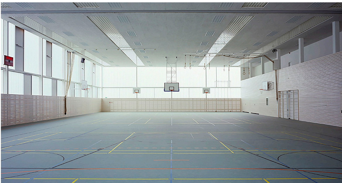
The building envelope of this ball sports complex in Ingolstadt, Germany, by Fink+Jocher, consists of a channel glass construction filled with translucent thermal insulation between its two glass profile shells. This enables sufficient light to enter without causing disruptive shadows on the court.
